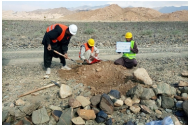
Survey in progress for feasibility study and preliminary design of Roads, Quetta Zone/Quetta Cluster, Balochistan
