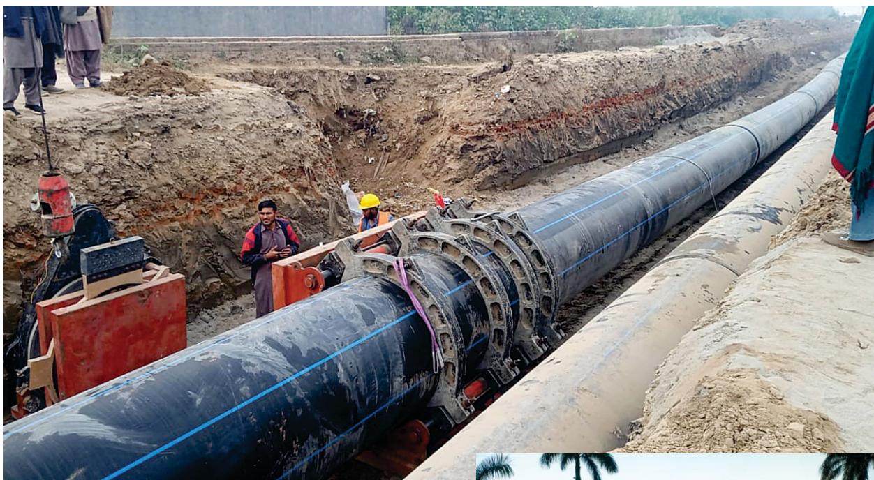
Laying of force main under way in Sialkot under Punjab Intermediate Cities Improvement Investment Program (PICIIP), Package-2
