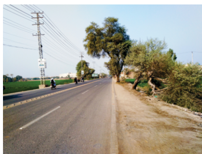
Multan Ring Road Project site
