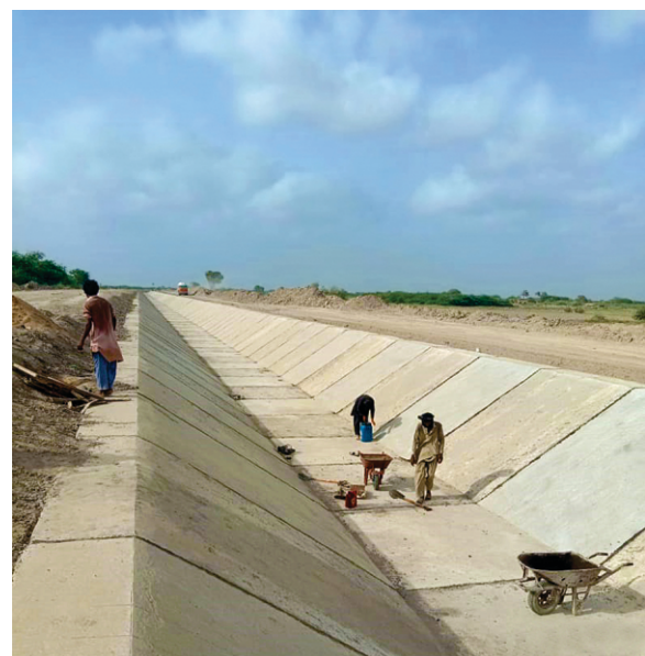
Work in progress for cement-concrete lining of Otero Lal Branch Canal Project, Sindh
