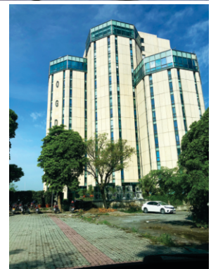
Front view of Oil and Gas Development Company Ltd. Head Office, Islamabad
