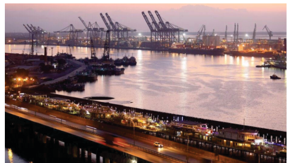
Dry Bulk Clean Cargo Terminal, East Wharf, Karachi Port
