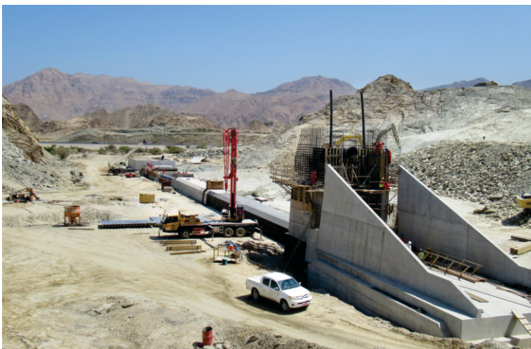
Construction of intake tower and stilling basin in progress for main Al-Jufainah Dam, Sultanate of Oman
