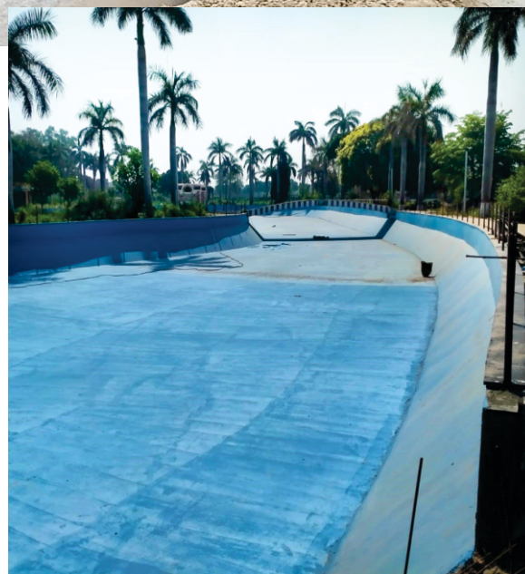
Lake coating at Gulshan-e-Iqbal Park in progress in Sialkot under PICIIP, Package-2
