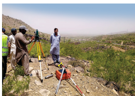
Widening and strengthening of Rakhi Gaj-Bewata Package, Punjab
