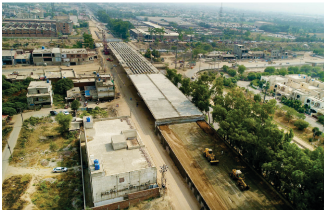
Launching and pouring of deck slab over flyover at Shahkam Chowk, Lahore
