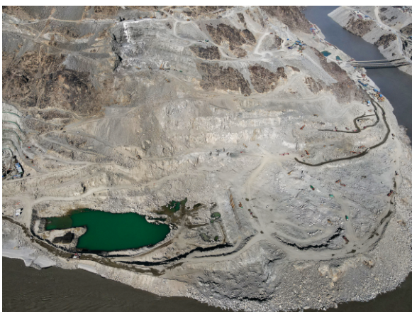
A view of Diamer Basha Dam Project right abutment and diversion canal
