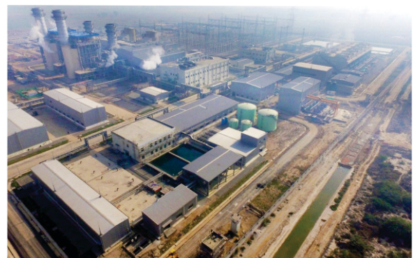
An aerial view of 1,180MW RLNG-based CCPP at Bhikki, Sheikhpura
