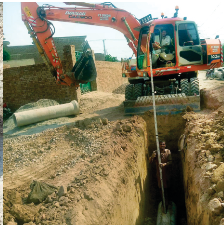
Construction works in progress for 12 Annual Development Programme (ADP) Schemes by WASA, Multan
