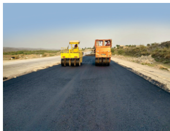
Construction activities under way for Dualisation and Improvement of Pindigheb-Kohat Road
