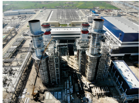
An aerial view of 1,263MW Regasified Liquefied Natural Gas (RLNG)-based Combined Cycle Power Plant (CCPP) near Trimmu Barrage at Haveli Bahadur Shah, District Jhang
