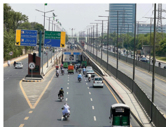
Construction of Underpass at Gulab Devi Hospital and additional lanes on Lahore Bridge
