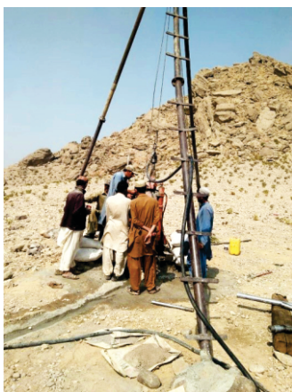
Geotechnical investigations under way for Murunj Dam Project, District Rajanpur
