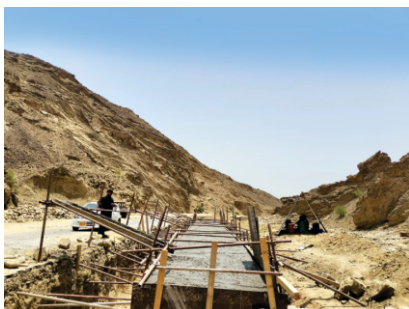
Work under way for Jhaljao-Bela Road Project in Balochistan
