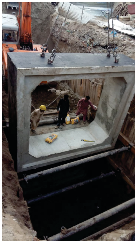
Laying of precast conduits in progress for Haji Camp-River Ravi Stormwater Drainage System, Lahore
