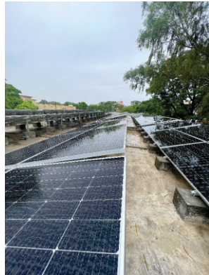
Installation of solar panels in District Gujrat Hospital for Solarisation and Retrofitting at 13 Punjab Hospitals Project
