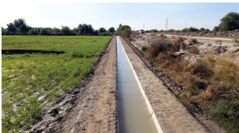
A watercourse lined under Gomal Zam Dam Command Area Development and On-farm Water Management for High Value and High Efficiency Agriculture Project, Khyber Pakhtunkhwa
