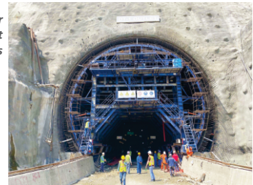
Diversion tunnel for Mohmand Dam Project in progress
