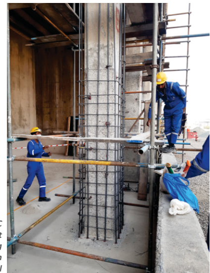
Preparation of RC column jacket at site for the Cooling Tower Rehabilitation Works, Khanewal
