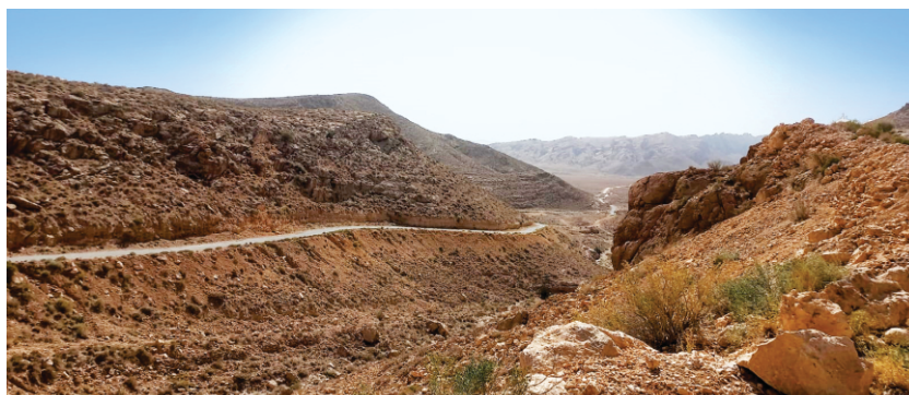
Kalat-Pindran Road Project, Balochistan
