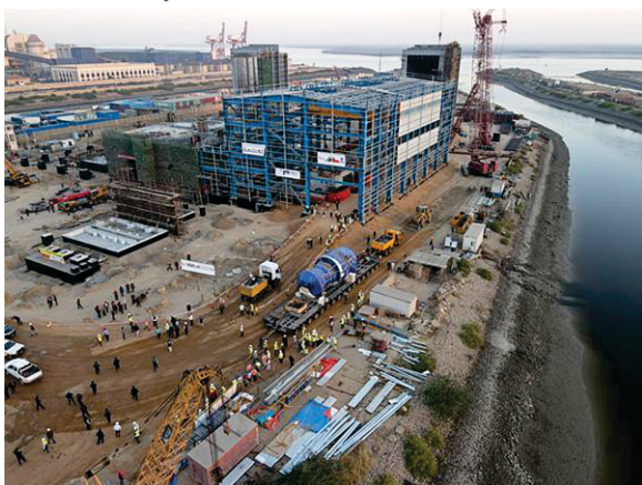
Construction work in progress for 900MW Bin Qasim Combined Cycle Power Station and associated Projects
