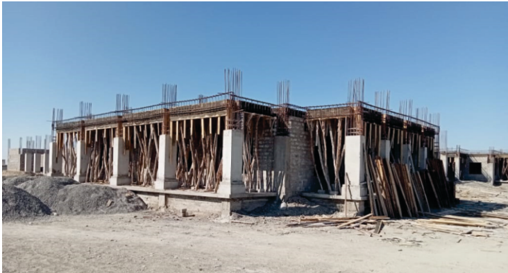
Under-construction Balochistan High Court Complex, Turbat
