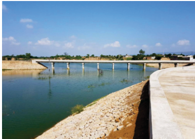
A bridge constructed at Chak Baqar Shah for Arrar Mughlan Dam under Annual Development Programme (ADP) Irrigation Projects
