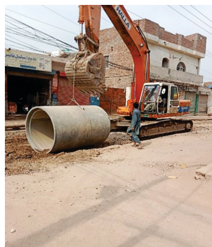
Site activities under way for Replacement of Outlived Sewer in Multan, Phase-II
