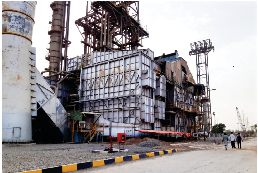
Cold-leg hot-leg refractory equipment structure being strengthened for structural capacity enhancement requirements at Fatima Fertilizer Company Ltd., Rahim Yar Khan
