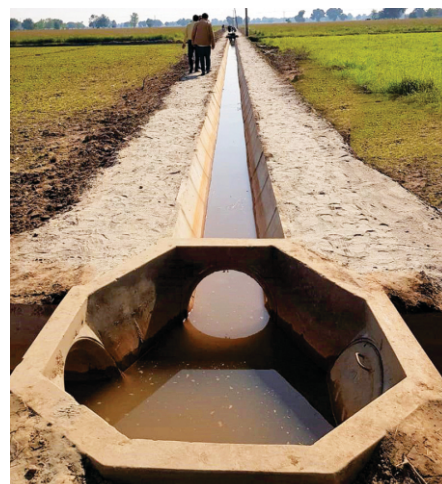
A watercourse lined under National Program for Watercourses' Improvement in Pakistan, Phase-II
