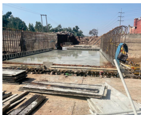
Construction of an aqueduct across Bara River for the Warsak Gravity and Lift Canal Project
