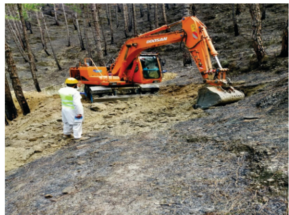
Site activities in progress for 500 kV Transmission Lines interconnection arrangement for power evacuation from Suki Kinari, Kohala and Mahl Hydropower Project
