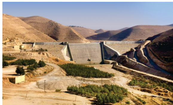
A view of Wala Dam, Kingdom of Jordan, after raising
