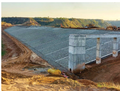
A view of under-construction Mohatta Dam in District Rawalpindi for ADP Irrigation Projects
