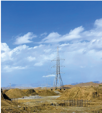
220 kV Double Circuit Transmission Line on Rail Conductor from Dera Ismail Khan in Khyber Pakhtunkhwa to Zhob in Balochistan
