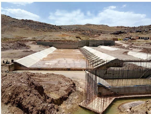
Construction work for Ahmad Zai Weir Structure for the Balochistan Water Sector Development Project
