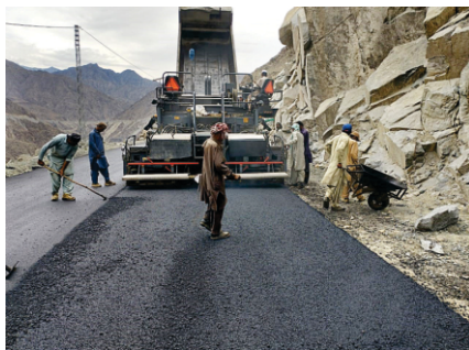
Construction works in progress for Shatial-Thor Nullah Bypass
