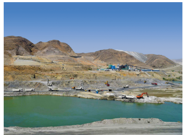
Cutting/excavation of re-regulation pond for Mohmand Dam Project
