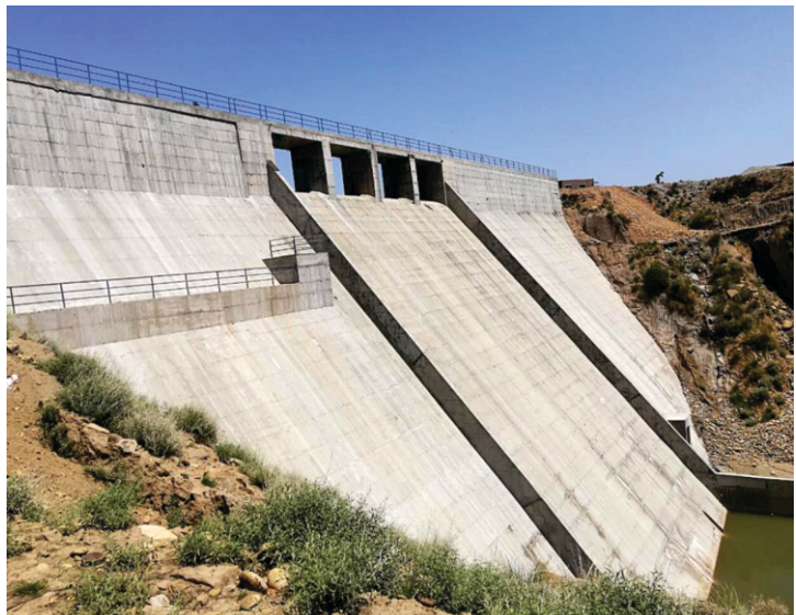
A view of Pandori Dam in Jhelum District under ADP Irrigation Projects
