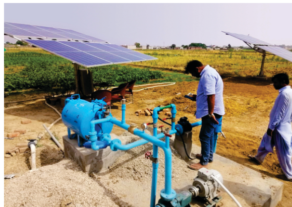
Work in progress for drip Irrigation system coupled with solar system under Promotion of High Value Agriculture through Solarisation of Drip and Sprinkler Irrigation System
