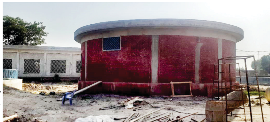
Finishing works of pump house in progress for Augmentation of Disposal Station, Multan
