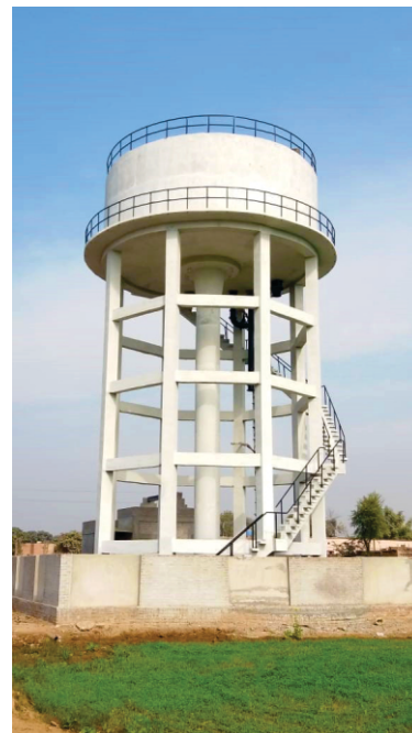
Work under way for Five ADP Schemes (2017-18) of WASA, Multan
