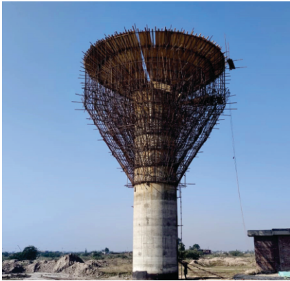
Construction of overhead reservoir in progress at Quaid-e-Azam Business Park site, Sheikhupura
