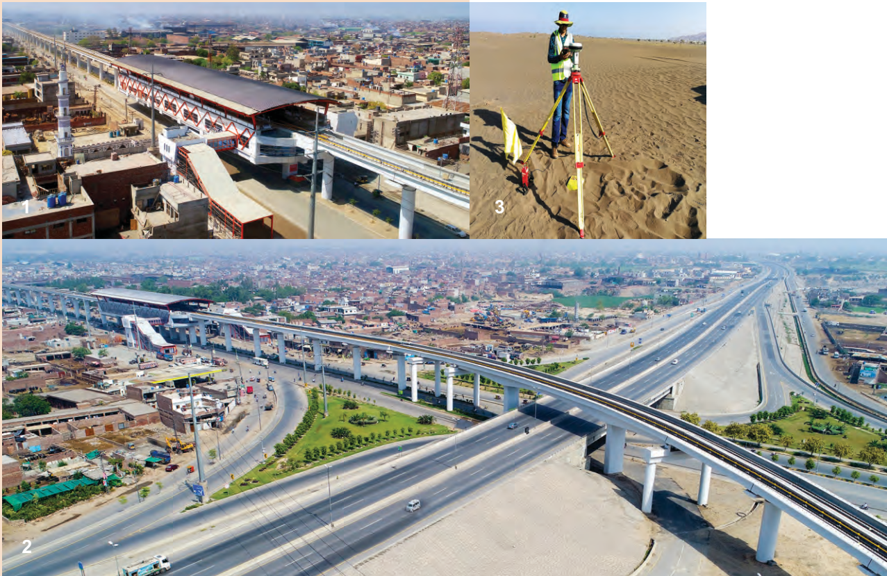
3. Work in progress for Roads in Al-Sahil Area, Wilayat Quriyat, Oman
