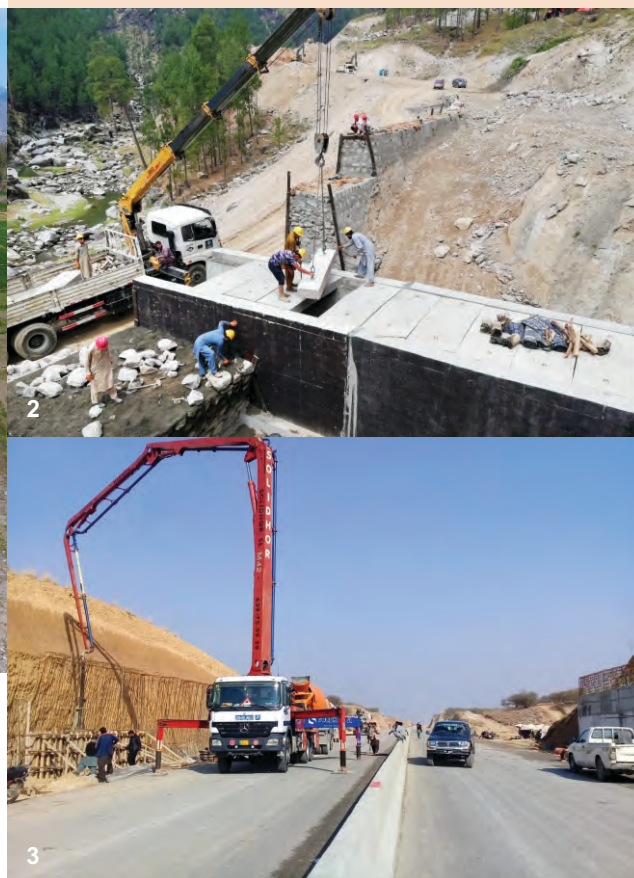
1&2. Two different views of the under-construction Havelian-Thakot Road Project for the China-Pakistan Economic Corridor
