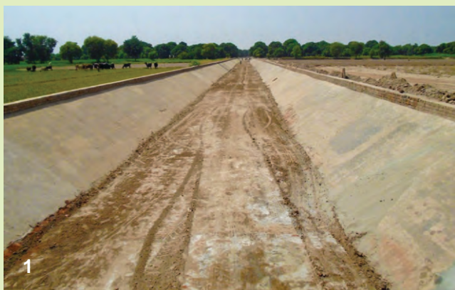
1. A view of the completed brick-lined Sullage Carrier Project under the Prime Minister's Package, Multan
