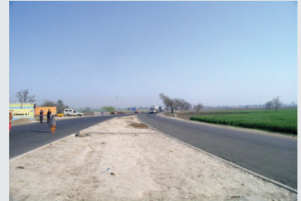
A view of the completed Khanewal-Lodhran Road Project
