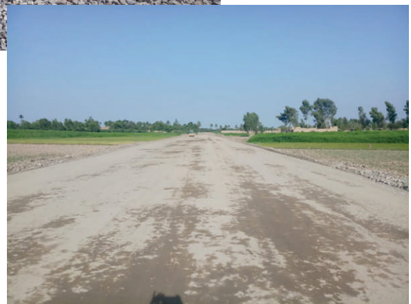
Natural ground compaction for the Circular Bypass Road, Bannu
