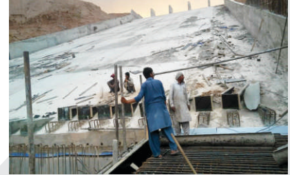
Construction of Mujahid Dam spillway under the Mega Irrigation Projects in Punjab
