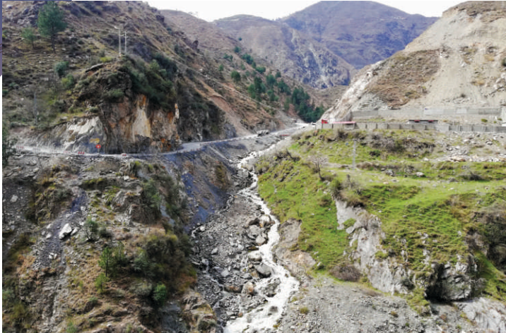
A view of the route for 500kV Transmission Line for power evacuation from Suki Kinari, Kohala and Mahl Hydropower Projects in the Northern Areas of Pakistan
