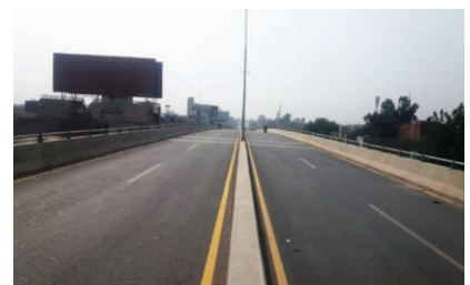
Overhead Bridge at the Depalpur Chowk, Okara
