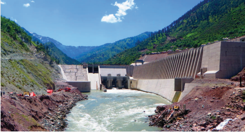
The upstream view of diversion dam spillway for the 969MW Neelum-Jhelum Hydroelectric Project in Azad Jammu and Kashmir
