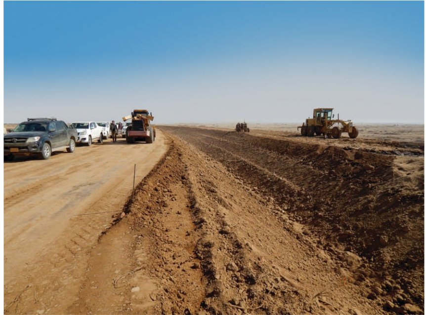
Work in progress for the K-IV Project, Karachi
