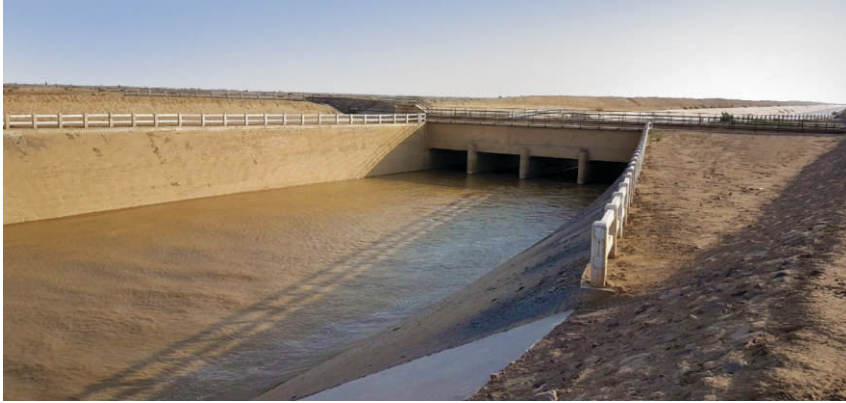
Syphon for the Kachhi Canal Project, Balochistan
