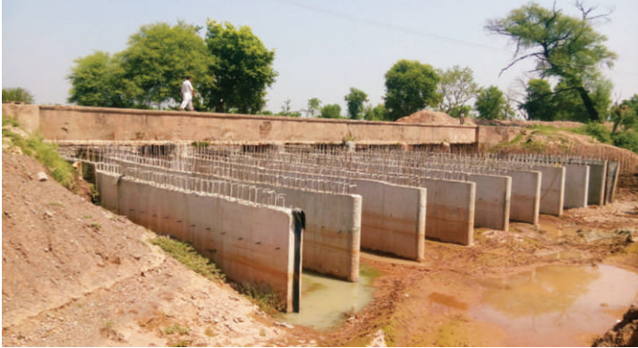
Under-construction drainage culvert for Remodeling of Warsak Canal System Project
