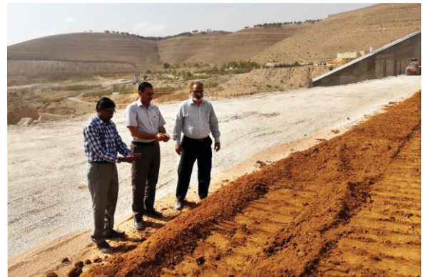
Site inspection for Raising of Walla Dam Project, Jordan
