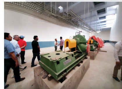
Site visit for Pre-Treatment System on the Left Bank Outfall Drain, Sindh
