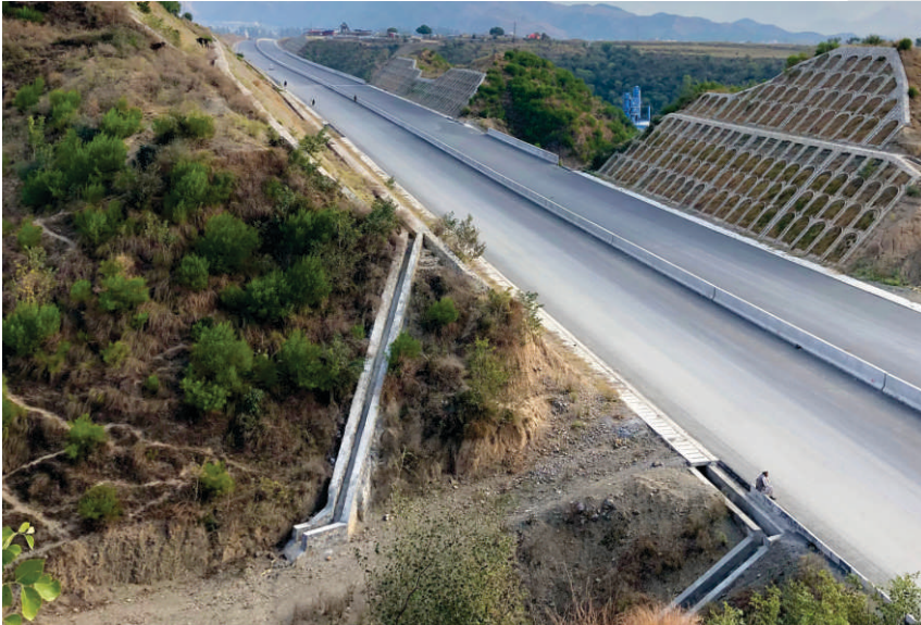
A portion of the Havelian-Thakot Section under China-Pakistan Economic Corridor (CPEC)
