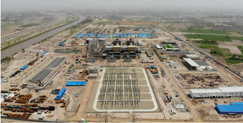
A panoramic view of 1263MW Regasified Liquefied Natural Gas (RLNG)-based Combined Cycle Power Plant near Trimmu Barrage at Haveli Bahadur Shah, Jhang
