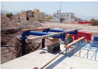
Water Distribution Networks for Nakhal, Awabi and Wadi Al-Maawil Wilayats in al Batinah Region (Phase-I), Oman
