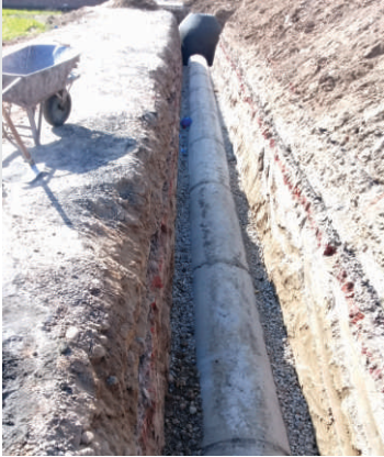
Laying of pipe under Five Water Supply, Sewerage/Drainage Schemes in Gujranwala
