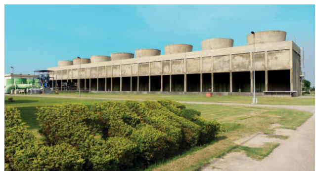
Rehabilitation of Cooler Tower building for the 450MW Combined Cycle Power Plant, Abdul Hakim, Khanewal for Rousch (Pakistan) Power Limited
