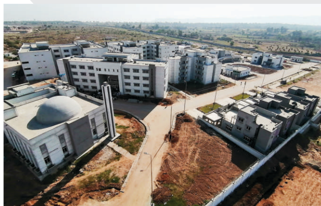
A view of Airport Security Force Camp under New Islamabad International Airport Project
