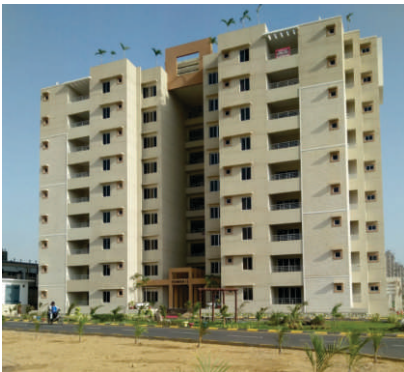
A view of residential towers-2 for Navy Housing Scheme, Karachi
