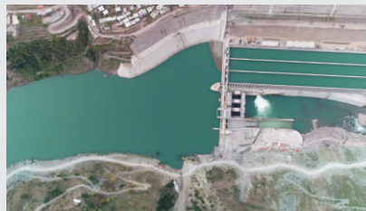
An aerial view of diversion dam for 969MW Neelum-Jhelum Hydroelectric Project
