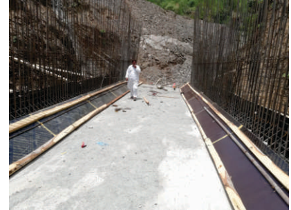
Construction work in progress for Abbottabad Bypass Road Project
