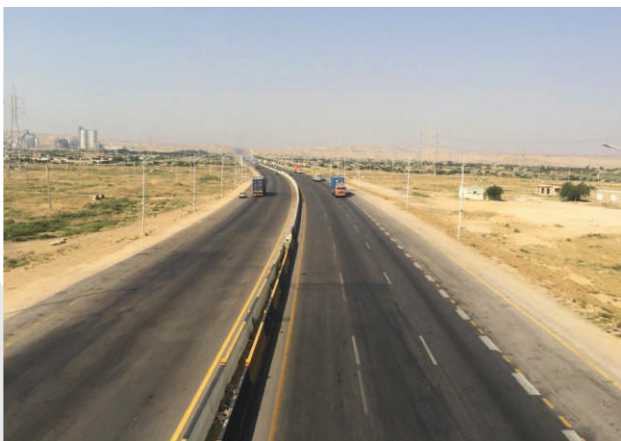
A view of the ongoing Karachi-Hyderabad Motorway Project
