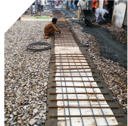
Work in progress for Provision of Clean Drinking Water, Sewerage System, PCC of Streets and Allied Facilities in Various Areas of Lahore Project
