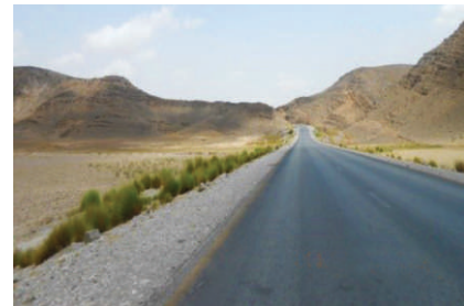
Work in progress on Khuzdar-Chaman Section of Karachi-Chaman Highway
