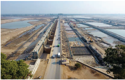
An aerial view of Panjnad Barrage
