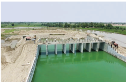
View of a head regulator constructed on Lala Creek of Indus River under Annual Development Programme Projects
