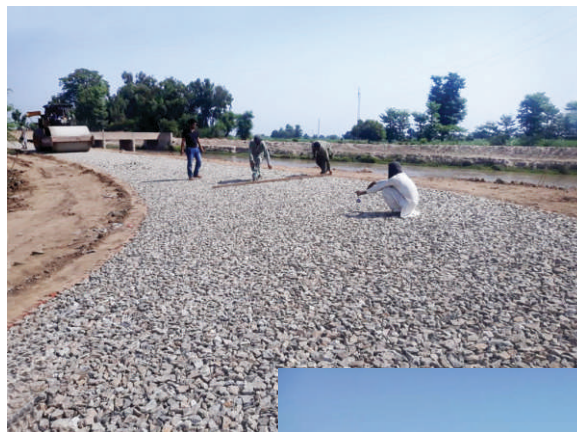
Work underway for Roads of Rural Accessibility Programme in Highway Circle 1 & 2, Faisalabad
