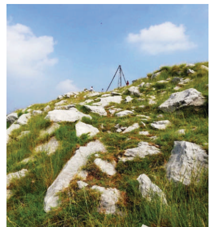
Borehole for coring in limestone quarry site for Haripur Cement Plant
