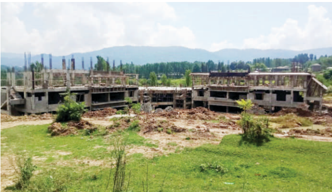
Under-construction girls hostel building at the Tarar Campus of the University of Poonch, Rawalakot, Azad Jammu and Kashmir
