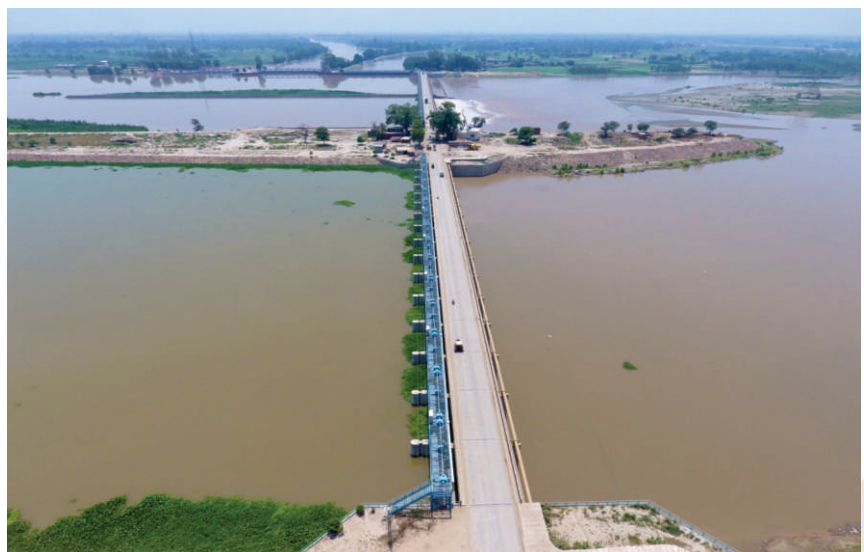
An aerial view of Balloki Barrage, gated spillway and canal head regulators
