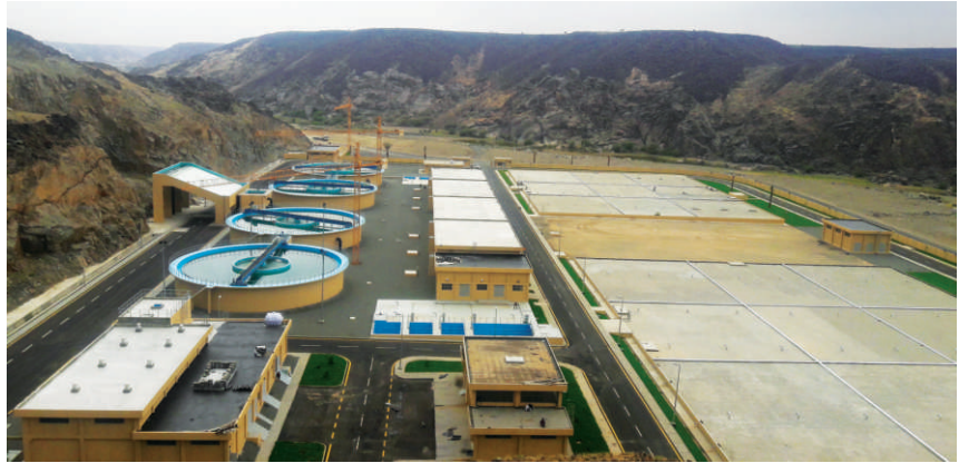
A water purification plant for Water Transmission from Khulais and Rabigh Dams to Jeddah Project, Saudi Arabia
