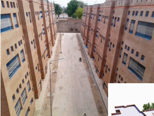
Main prisoner barracks constructed for the Central Prison Peshawar, Phase-I
