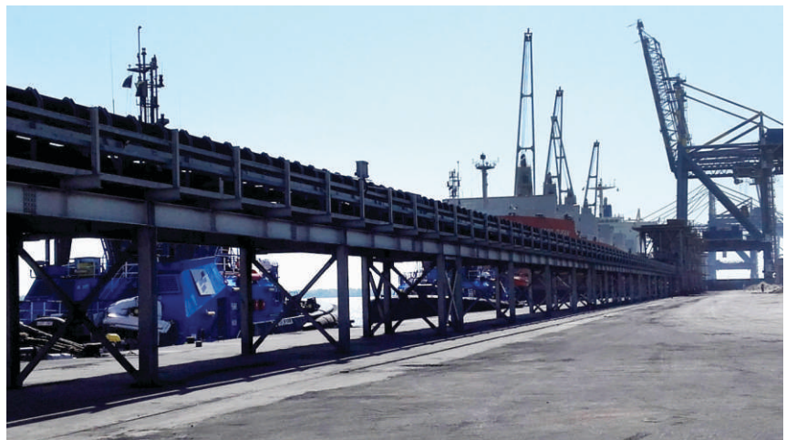
Work in progress for Conversion of Marginal Wharf Berths 3 & 4 into Coal Terminal at Port Qasim, Karachi
