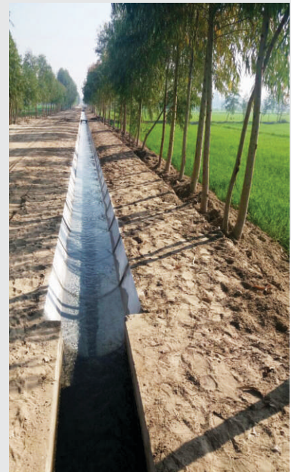
A lined channel under Optimising Watercourse Conveyance Efficiency through Enhancing Lining Length Project in Bahawalnagar, Punjab
