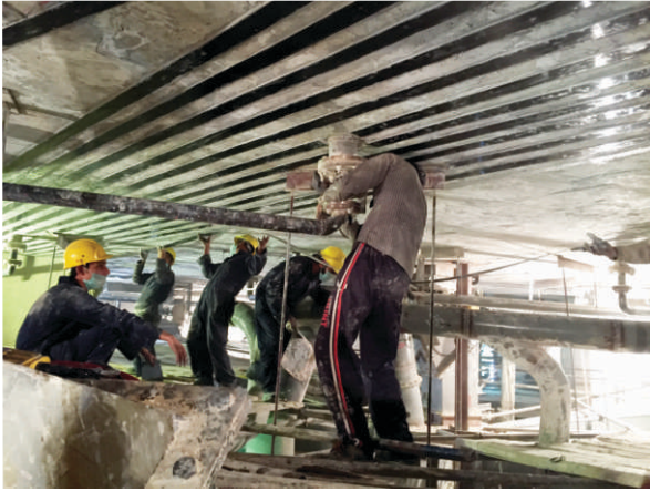
Repair work at Maple Leaf Cement Factory, Iskanderabad, Mianwali
