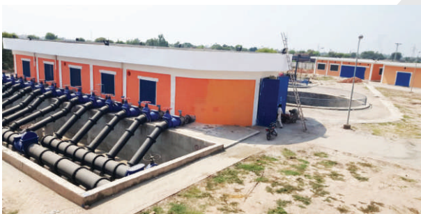
A pump house at New Shah Shams Colony under Prime Minister's Southern Punjab Package (Part-I) for improvement of water and sewerage systems in Multan
