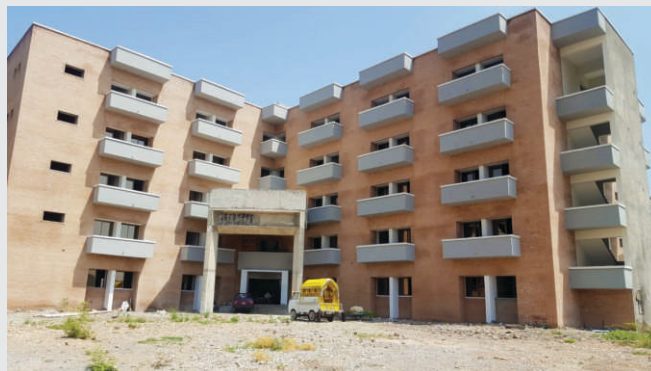
Under-construction Kohat Institute of Medical Sciences
