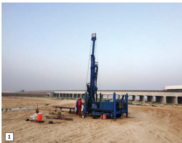
1. Work underway for dual carriageway road for NR-32, Phase-I, Duqm Town, Oman
