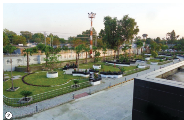
1&2. Views of the Expansion and Renovation Project of Bacha Khan International Airport, Khyber Pakhtunkhwa
