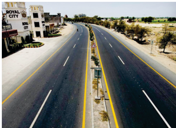
Recently completed section of the Sahiwal–Arifwala–Bahawalnagar Road
