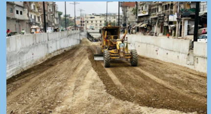
Construction activities in progress
