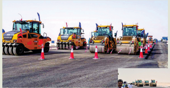
Work in progress on the Adam–Thumrait Road Project
