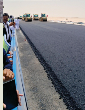
Work in progress on the Adam–Thumrait Road Project
