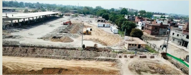
Construction activities in progress at the Data Darbar Redevelopment Project
