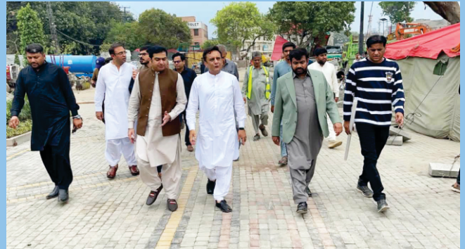
The Client along with other officials visiting the project site while construction activities are in progress
