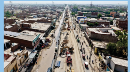
An aerial view of the project site
