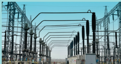
Augmentation Works of (02) Two sets of 220kV Circuit Breakers out of Six (06) completed at 220/132kV Summandari Grid Station
