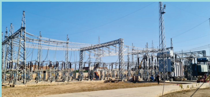
132kV Busbar strengthening works completed at 220/132kV Bannu Grid Station
