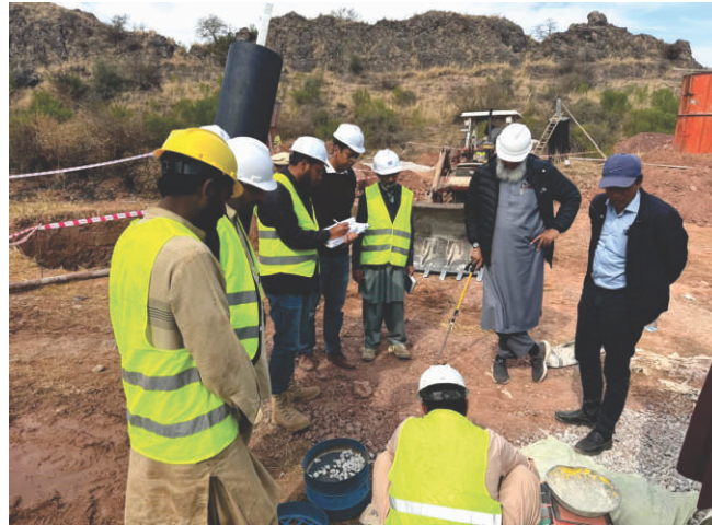
Field activities in progress at the project sites
