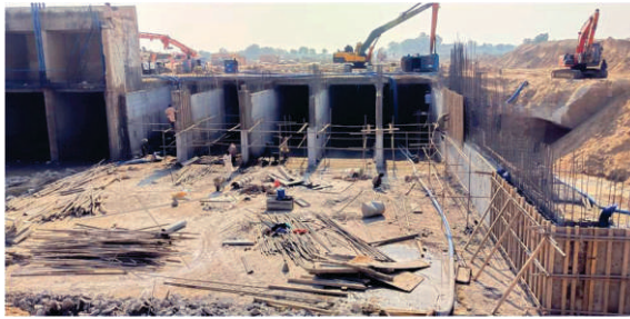
Work in progress at project site
