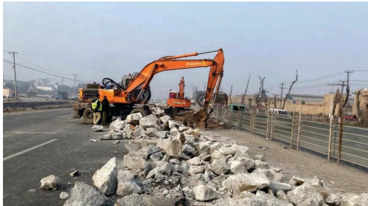
Work in progress at Gujranwala Mass Transit
