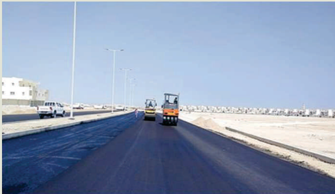
Laying of Bituminous Wearing Course
