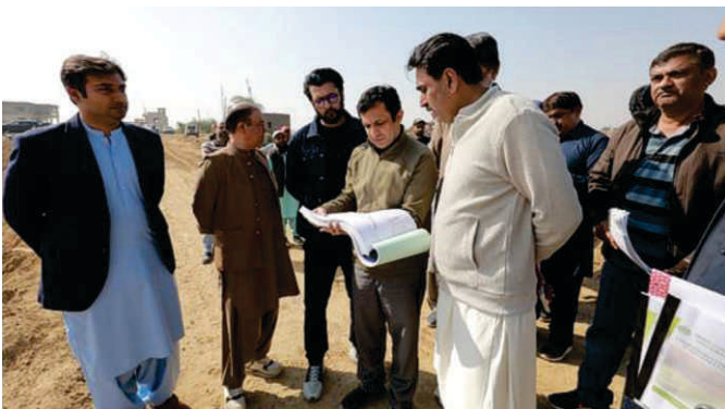
Minister of Irrigation and Planning Department, Government of Sindh, Mr. Jam Khan Shoro, and the Secretary Irrigation Department, Engr. Zareef Iqbal Khoro visiting the ongoing lining works on Kalri Baghar Feeder Upper Phase-1 Project.
