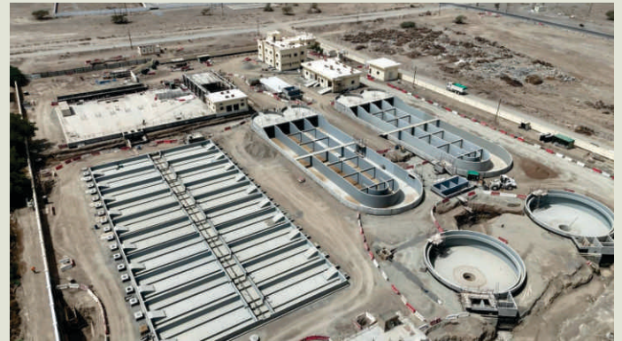
Sewerage Network and Sewage Treatment Plant, and Pipeline for Wilayat Al-Musannah
