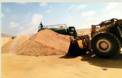
Disposal of blasting material
